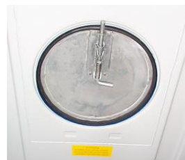
Figure 9.11 Roof hatch internal lock
