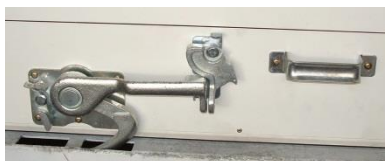
Figure 9.6 Roller shutter lock
